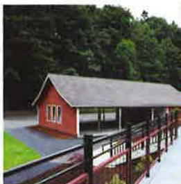
BEACH PARK PICNIC SHELTER
